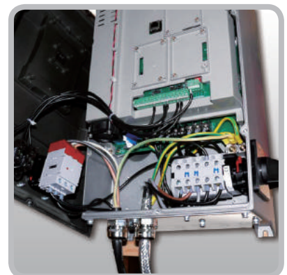
ROOM FOR BUILD-IN OPTIONALS
